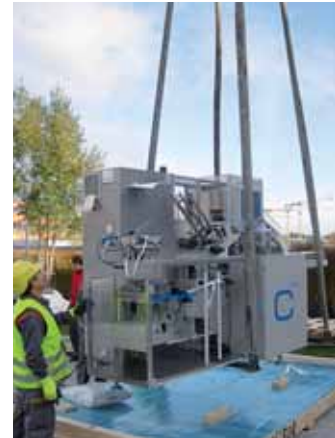
Tricky work with heavy lifting equipment: the cartoner and stretch-banding machine are brought into position, lifted over the front of the building and maneuvered into the production area. Technicians then completed installation.
